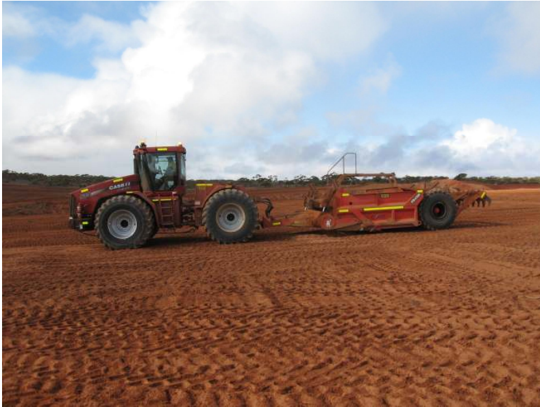
Fig.1. Carry grader at J-A, top soil stripped in foreground
