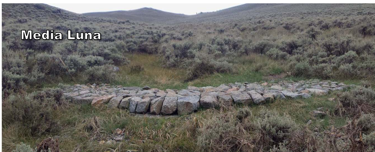
Figure 18. Media luna (looking upvalley) being used to spread sheet flow; note structure is placed on contour with uniform surface. Photo by: Shawn Conner
