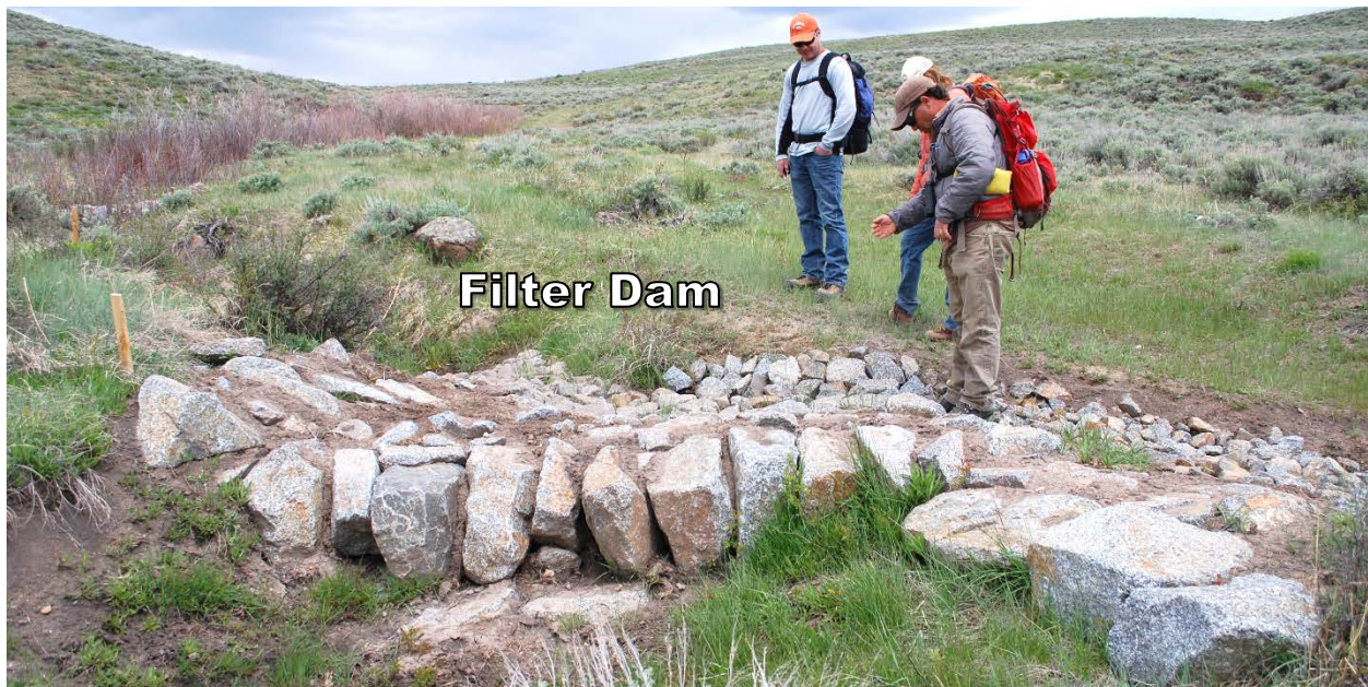
Figure 16. Filter dams temporarily impound shallow water but allow water to seep through the porous structure, thereby capturing sediment. Photo by: Betsy Neely DSC-0886
