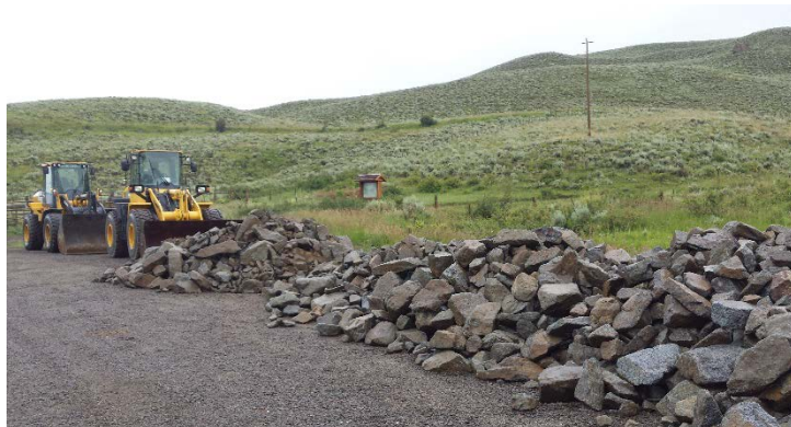
Figure 21. Staging rock for wheeled loaders to transport to restoration sites. Photo by: Shawn Conner
