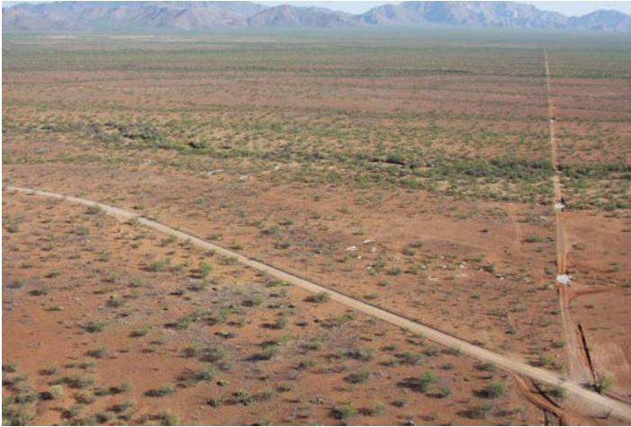
Figure 1. Aerial view showing intersection of Elkhorn Ranch and fence-line access roads.
