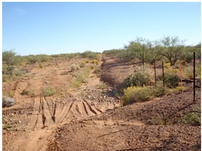
Figure 2. Incised fence-line road that triggered extreme watershed degradation at the Elk/LD Demo site.
